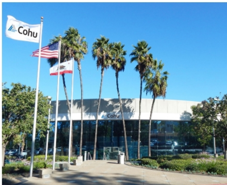
Cohu, Inc. Headquarters, Poway, CA
