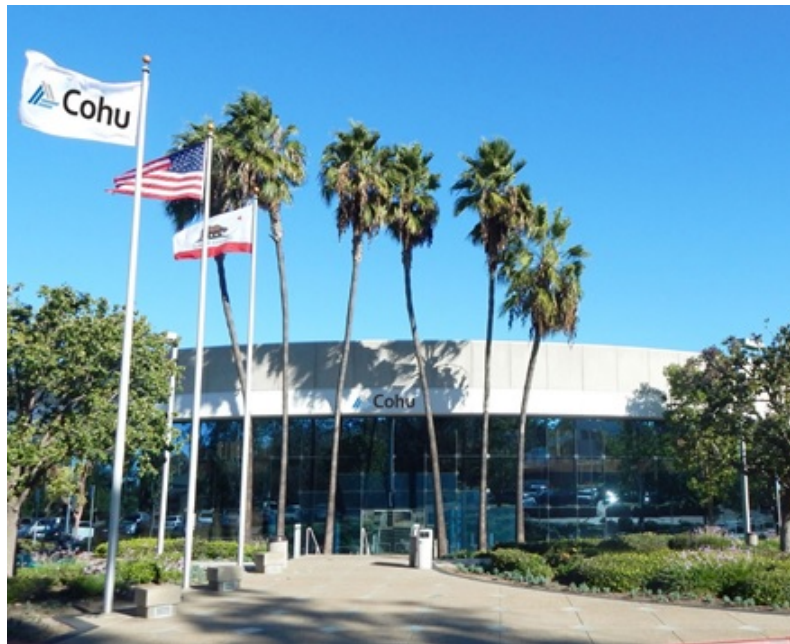
Cohu, Inc. Headquarters, Poway, CA
